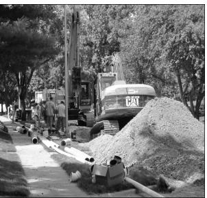
Work for phases includes in- Summer 2013 creasing the capacity of the storm water convevance in addition to separation of the storm and sanitary flows. The proiect includes design and construction of approximately miles of new storm sewer ranging in size from 15-inch diameter pipe to 12-foot by 10-foot box culvert.
